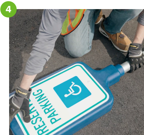
Slide the fully assembled 2-sided sign topper on to the post.
