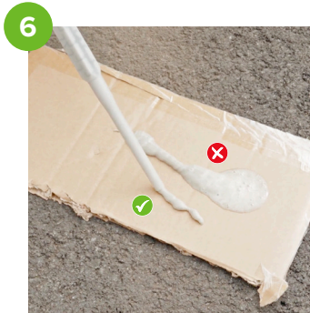
Dispense adhesive onto cardboard until the bead flows evenly.
