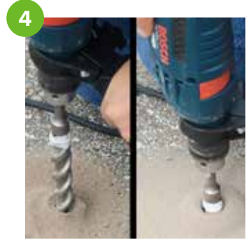
Drill 4 holes 7/8" diameter 6" deep.
