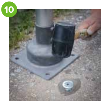
Using a rubber mallet, tap anchors into the holes until flush.
