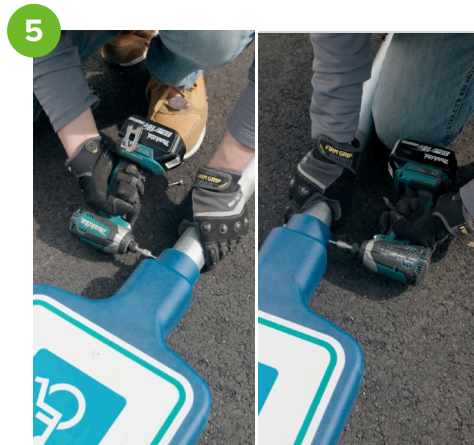
Secure the 2-sided sign topper to the post with the provided screws.
