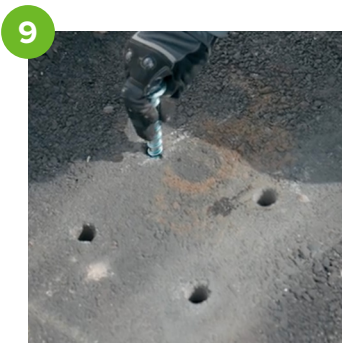
Insert anchors into hole by hand.
