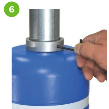
6 With the collar flush with the top of the bollard, tighten the set screw with the provided allen wrench.
