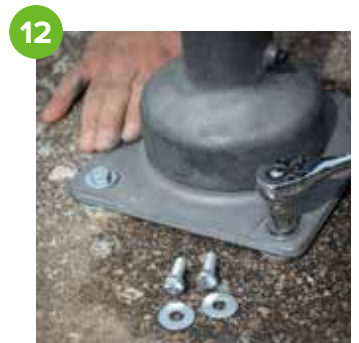
Using 9/16" ratchet, tighten anchors.
